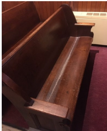
Cracked & Scratched Pews
